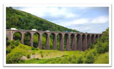
The viaduct runs across the Smardale Gill, and Scandal Beck, 27m high above the valley and was constructed of locally quarried sandstone featuring 14 arches of 10m span, over a total length of 170m.
