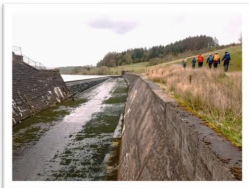
At the southeastern end of the dam, we cross a foot bridge over a spill way. Under normal circumstances this allows a gentle flow most of the time, as inputs via the Hodder typically exceed drawings by the treatments works. Have a look at the pictures from our 2022 walk to see how the infrastructure here looked when the water level was suppressed to enable building works to progress.
