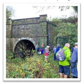
We remain parallel to the road for another 200m and then the path takes a sharp left turn — as indeed the canal once did. Ahead of us is a hill. When canals were built, there were three options for dealing with a hill, avoid by taking a circuitous contoured route around it, build locks (and a water supply to them) to take the canal up and over, or as was chosen here, bore a tunnel through it.
