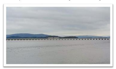
The viaduct itself was a significant challenge to build, and a novel construction method was developed to enable it to be built at lower cost and in a faster time; high pressure water jets were used to dig out the sand and silt below columns which were drawn down into the mud until they hit bedrock.
