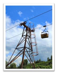
The shale is moved from the quarry to the brick works more than a mile away on the A683 using an aerial ropeway – the last surviving gravity powered ropeway in the UK. The system was built in 1924, and the remaining ropeway is one of two, originally constructed to serve the east and west works.
