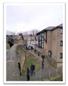
At the next bridge the towpath again changes side, and there is a "turning bridge" – a canal structure designed such that horses towing the boats could swap sides without unhitching the tow line.
